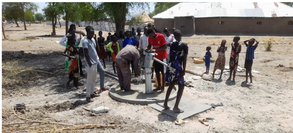
Borehole drilled by Caritas Malakal in Jonglei State in 2023
